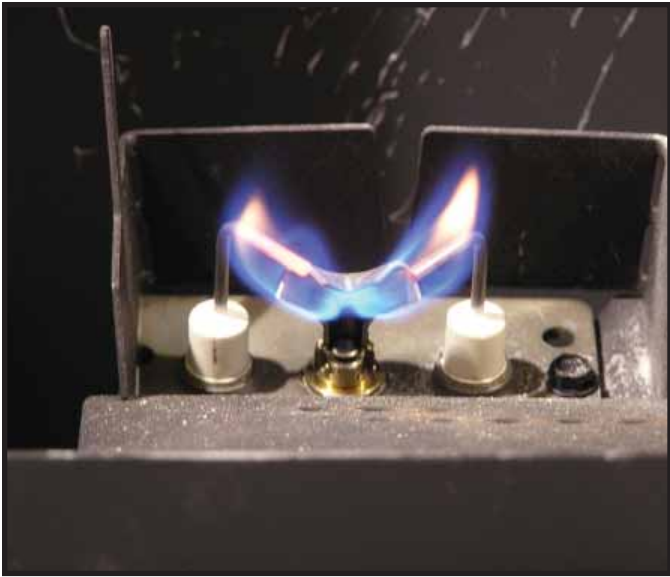
Figure 3.1 IPI Pilot Flame Patterns
